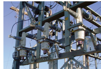
Retrofit installation with "Z"-shaped module Viper-ST on individual frames.
