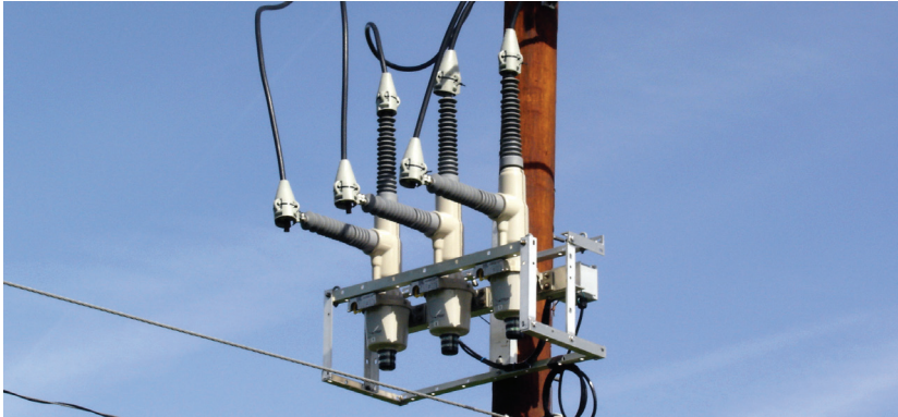
15kV center polemount Viper-ST
